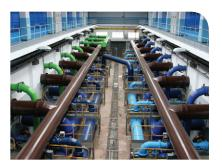
The water from WBMWD is treated at the MWD Weymouth Treatment Plant using conventional treatment methods, which include coagulation, flocculation, sedimentation and filtration. The water is then disinfected to kill any microorganisms, such as bacteria, and reduce the potential for their regrowth in the distribution pipes.
